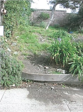
Wooden Retaining wall weakly supporting agapanthus to be replaced.
