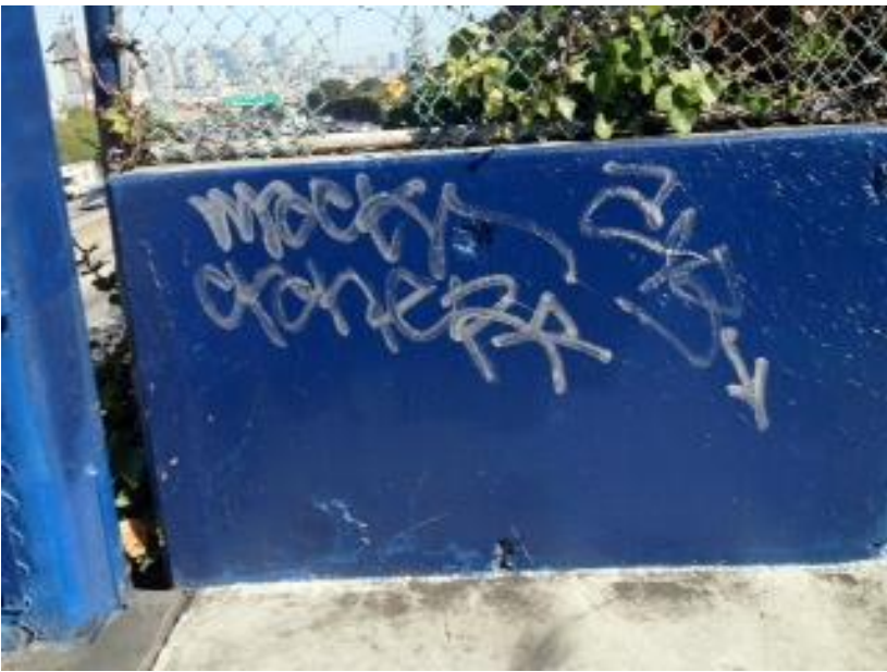
Thursday am Oct 27 looking north on east side
